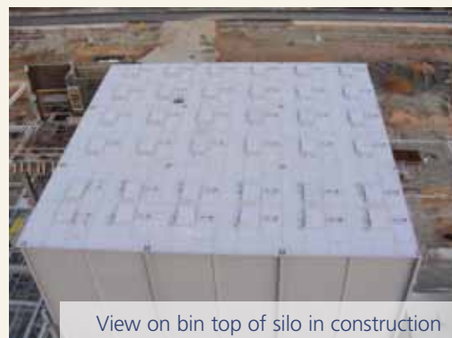
SCE's modular construction form
